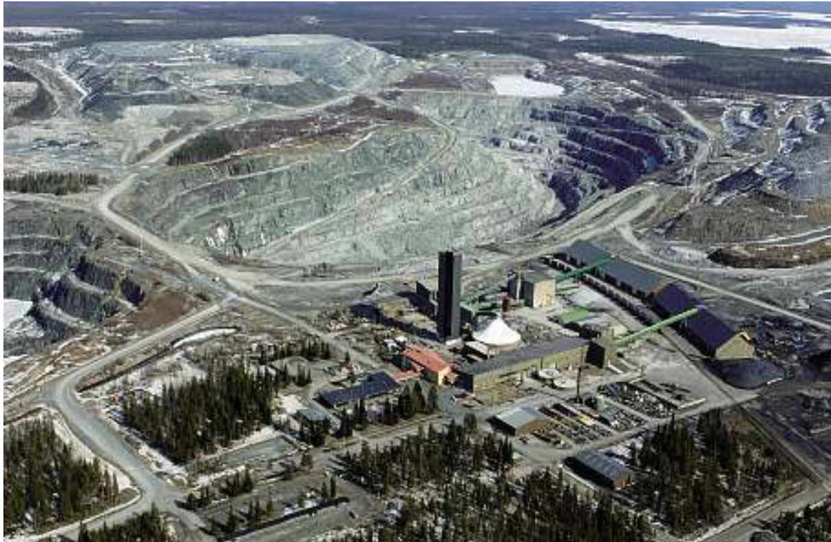
Fig. 11. Aerial photo of the Kemi open pit.
