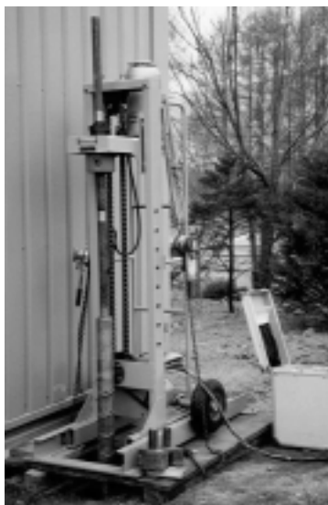
Figure. 6. View of the shallow-depth boring machine.
