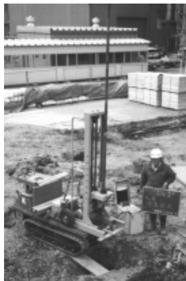
Figure. 7. Shallow depth boring machine mounted on a mini-caterpillar.
