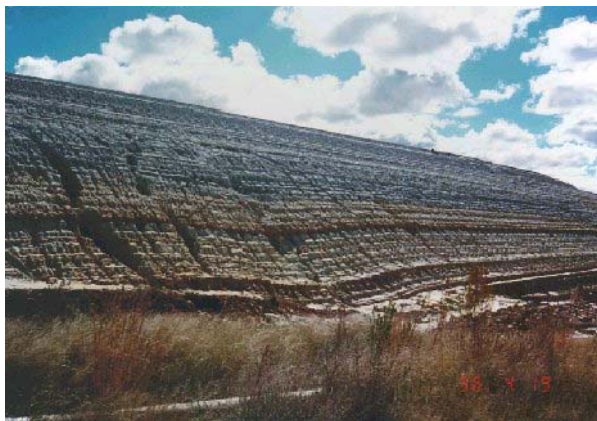
Subsidence under tailings dam wall due to sinkhole formation induced by mine dewatering. West Rand mining district, South Africa
