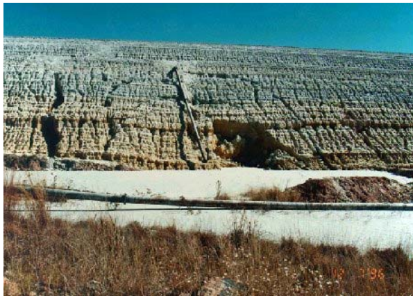
Tailings dam wall slump risk – West Rand mining district – South Africa)
