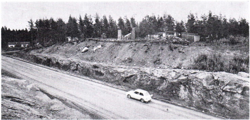
FIG. 4. Esker deposits resting on glacially sculptured bedrock. This kind of esker contains no ground water. Siltakylä, Pyhtää.
