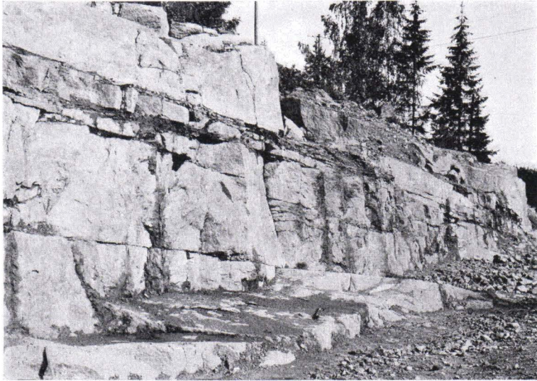
FIG. 14. The strong fracturing of rapakivi enables water to collect in the bedrock. Two vertical fracture planes at right angles are intersected by strongly developed horizontal planes. Ahvenkoski, Ruotsinpyhtää.
