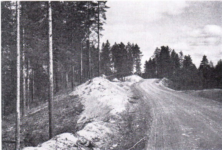
FIG. 12. Road leading to Murtoi runs across summit of dune 45. More gently sloping northwestern flank of formation appears at left in photo.
