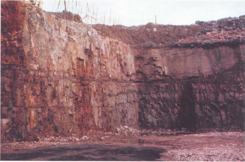
Fig. 15. The blasted southern (at right) and eastern (at left) walls of the Tahkoluoto harbour basin. Note the basal bounding surface of a SSE-NNW directed channel in the southern wall near the corner and corresponding large-scale cross-beds in the eastern wall.
