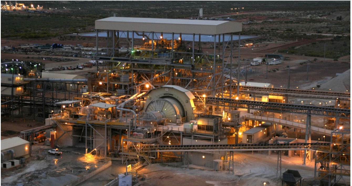
Figure 28. A mineral processing plant in the Southern Hemisphere (Source: Dee Bradshaw)
